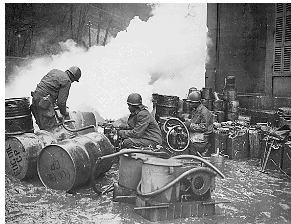
Soldiers of the 161st Chemical Smoke Generating Company, U.S. Third Army, move a barrel of oil in preparation to refilling an M-2 smoke generator, which spews forth a heavy cloud of white smoke. These men are engaged in laying a smoke screen to cover ferrying operations across the Saar River near Wallerfangen, Germany. December 11, 1944. Rothenberger. 111-SC-197552. (afri031.jpg)
